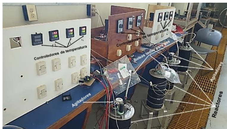
Figura B.3 Paneles de control
