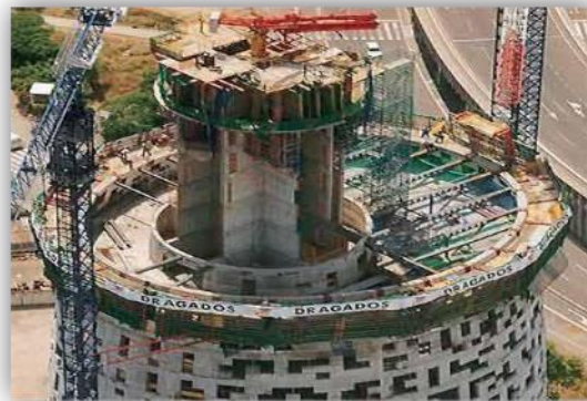
Fig 1.19 Torre Agbar (Argila, 2018).
