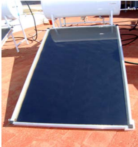
Figura 1.1 Colector solar plano
